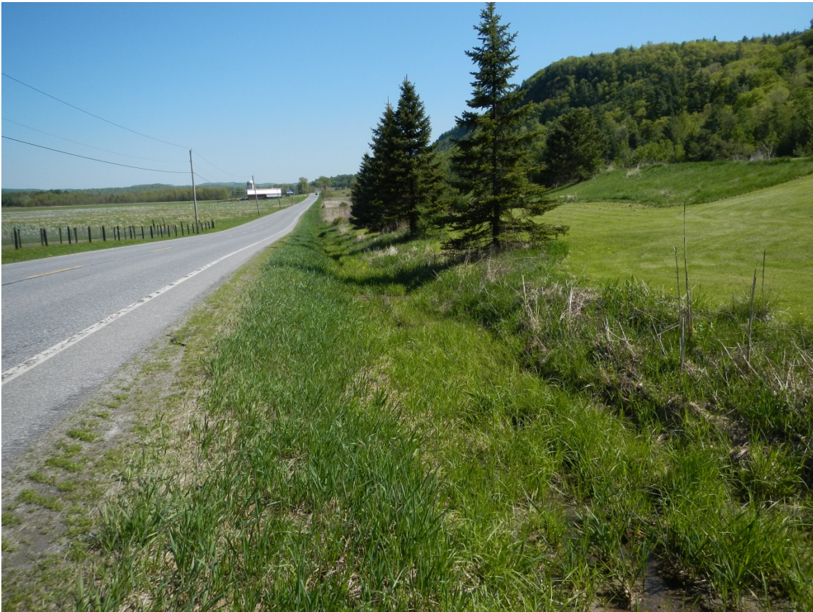
Photo 7. Typical NECPL cable route on Route 22A in West Haven, VT
