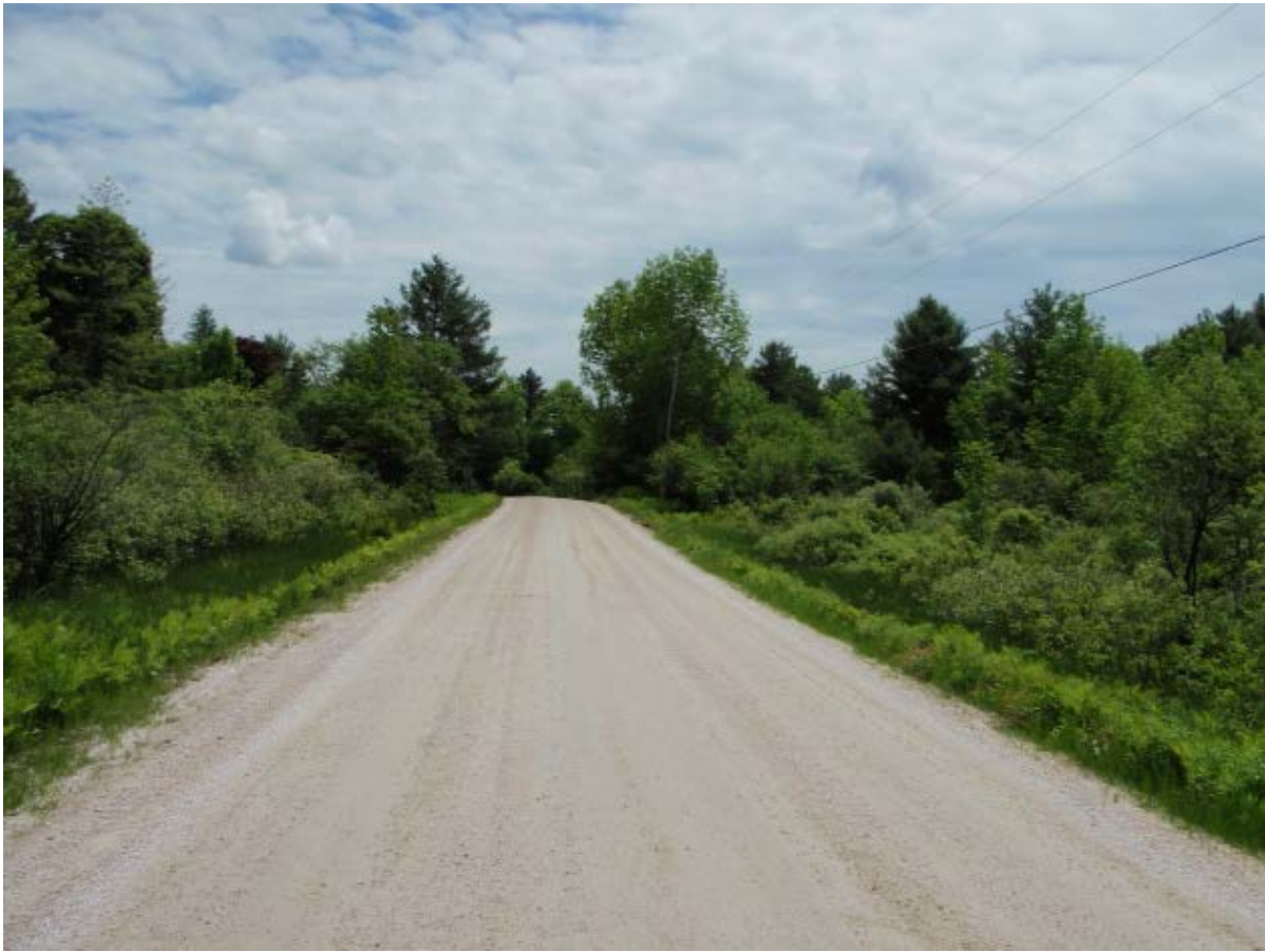
Photo 13. Typical NECPL cable route on town road in Ludlow, VT
